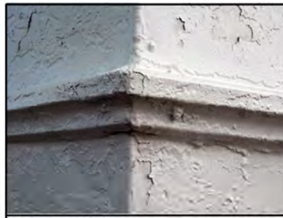
Historic paint layers on only joint in metal tower base wall
