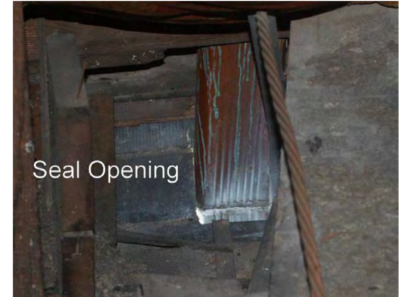
5- Seal Opening Between Downspout and Metal Fascia
