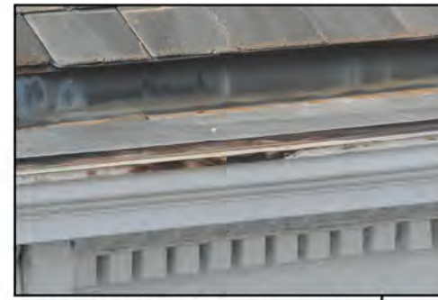
Rusting connection between original entablature and new gutter
