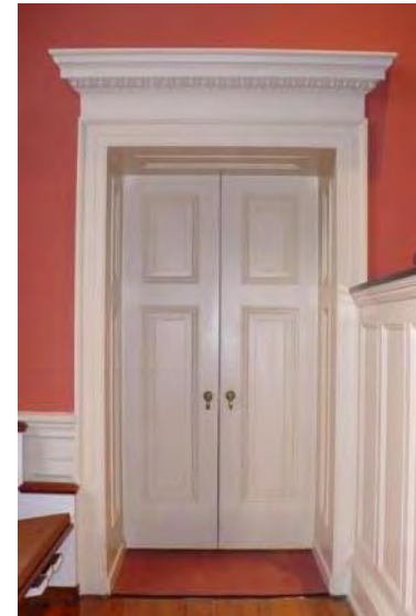
Door 105 seen from Sanctuary
