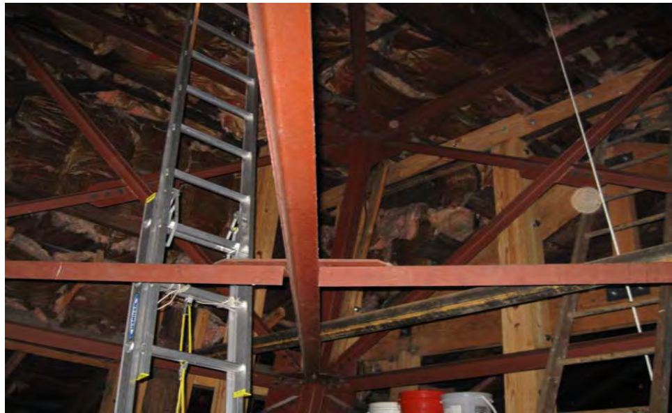
Photo 5 – Lower steeple support frame
