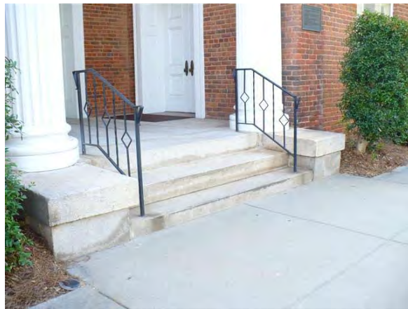
Sidewalk at main entrance to Sanctuary
