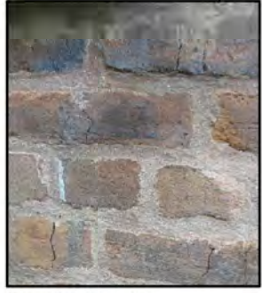
Cracked bricks
