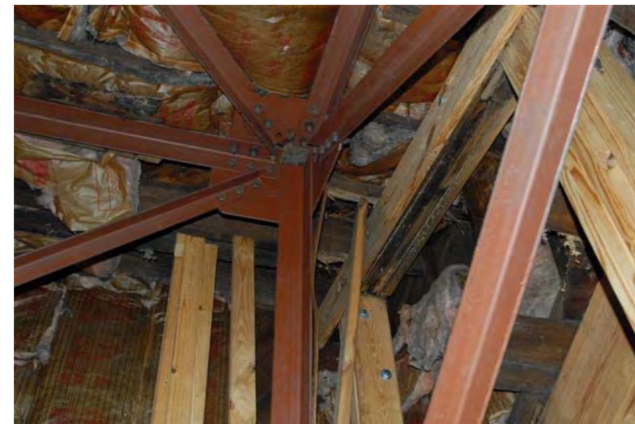
1970's Steeple steel support frame and recent wood frame intervention.
