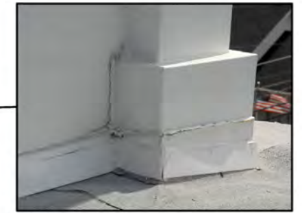
Flashing at corner base
