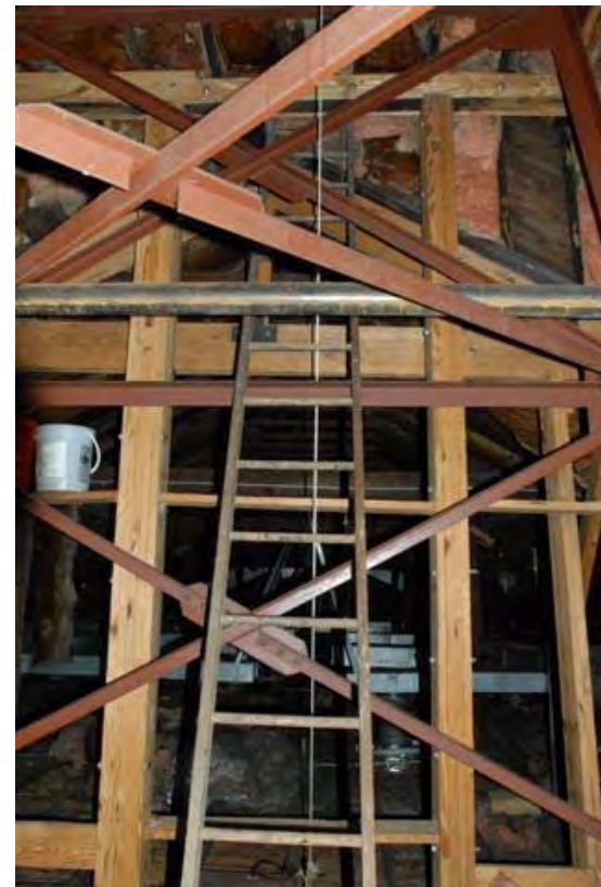
Additional structural support for belfry floor rafters
