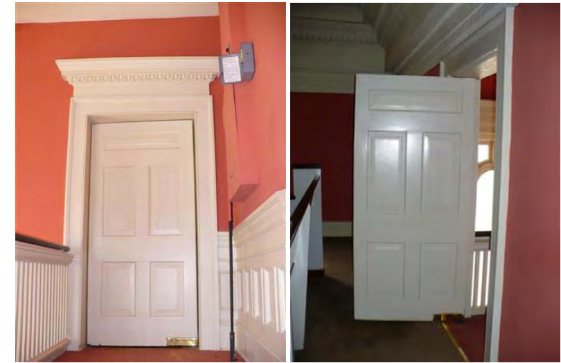
Door 202 seen from South Stair
