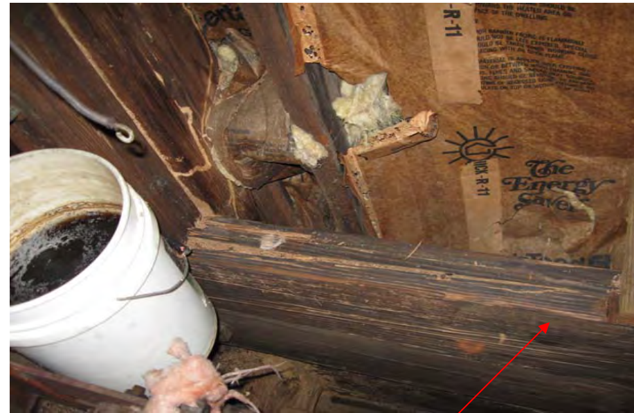
Photo 13 - Gable End Wall Framing (Base of Wall)
