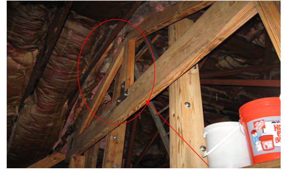
Photo 10 – Additional wood framing members for roof support
