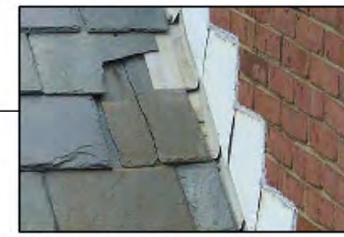
Falling/ missing slate repair
