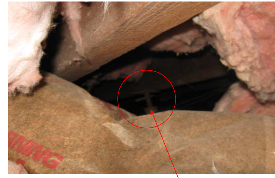
Photo 4 – Adjustable steel post for floor joist support
