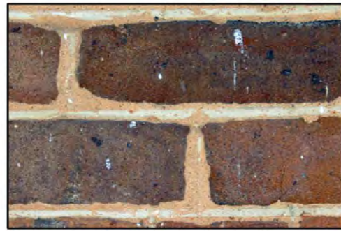
Remnants of paint or mortar coating
