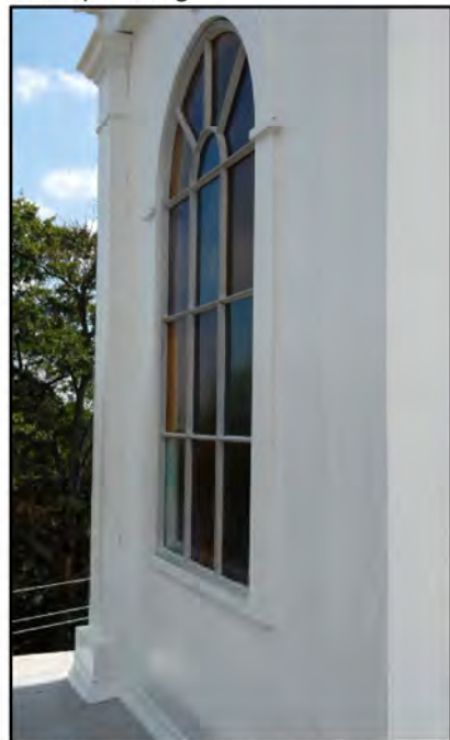
Colored glass window at North and South elevations
