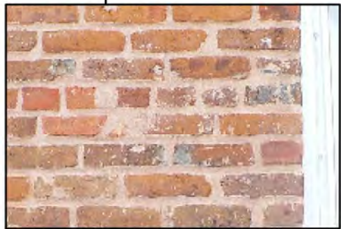
Overpointed- all voids filled with 1979 mortar
