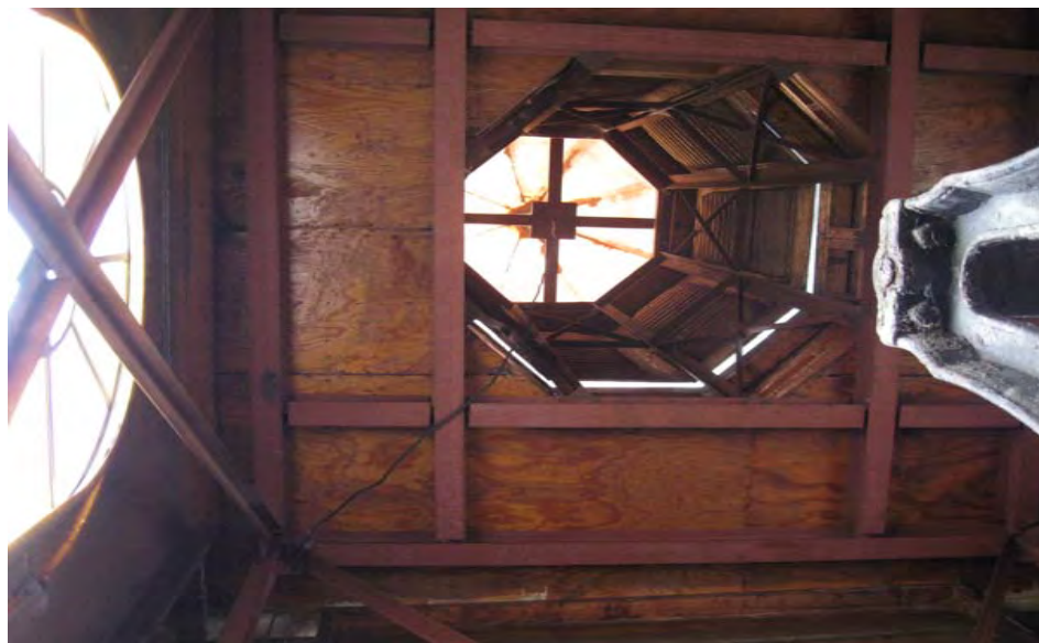
Photo 6 – Upper steeple support frame
