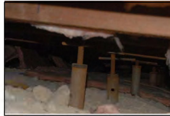
Typical steel jacks to support floor joists at midspan.
