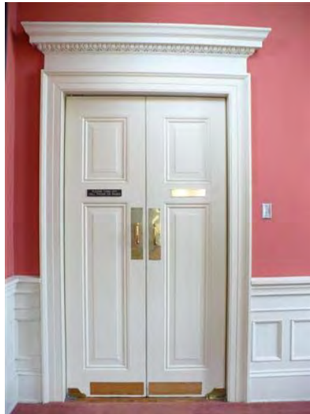
Door 103 seen from Stair Vestibule
