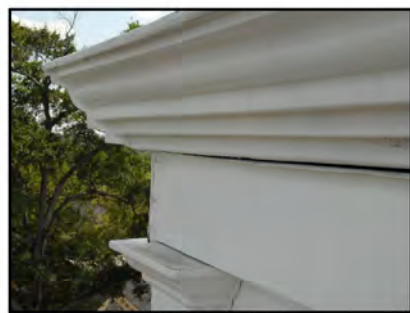
Cornice and frieze detail
