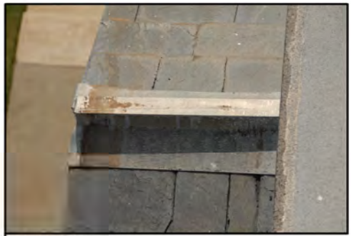
Galvanized steel ridge cap
