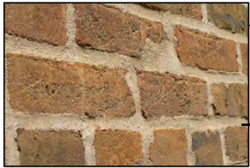
Scratched/ scored masonry
