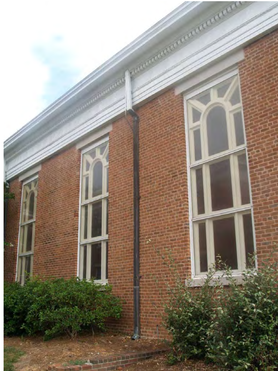
17 Rain Downspout – All Appear To Be In Good Condition
