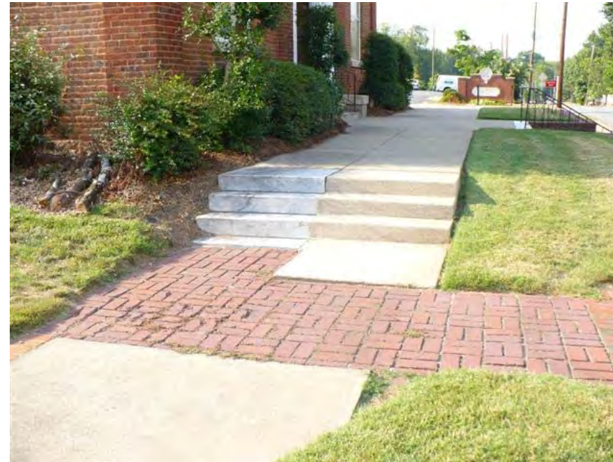
Double material steps: marble and concrete
