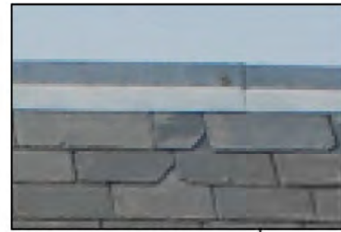
Chipped slate edges near galvanized steel ridge cap
