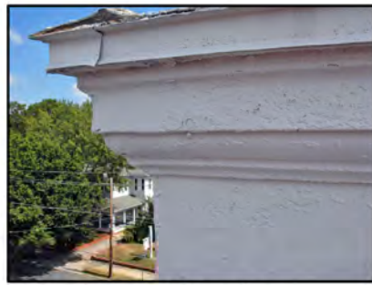
Tower base metal cornice
