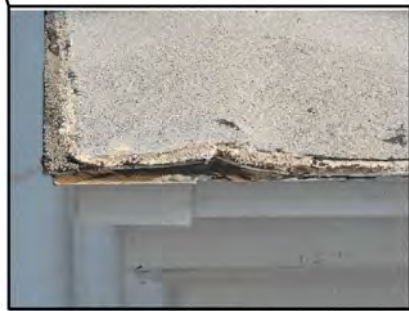
Edge of built-up roofing
