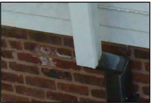
Efflorescence
