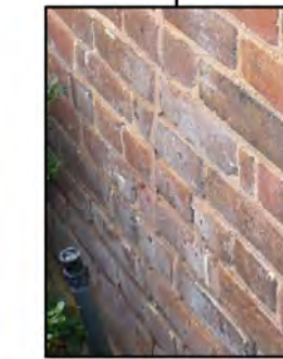
Efflorescence
