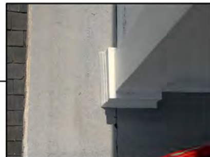
Built-up roofing and base
