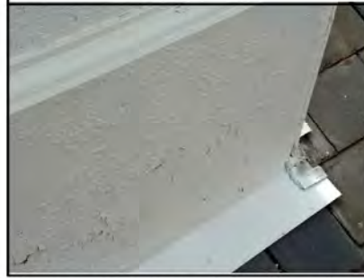
Flashing at slate roof (Northwest corner)
