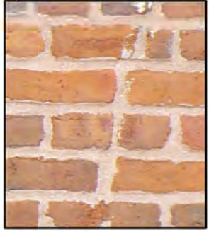
Overpointed brick repair (1979)
