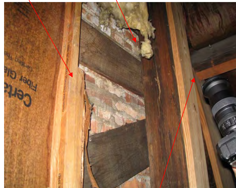
Photo 14 - Gable End Wall Framing (Reinforcement)
