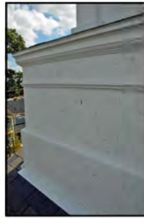
North side of tower looking West
