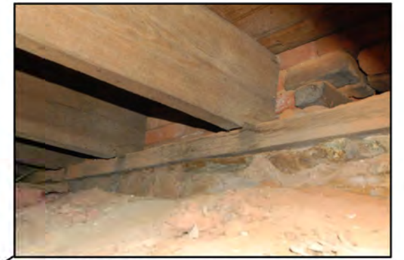
Floor joists sitting on top plate on granite foundation wall
