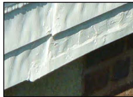
Metal entablature repaired with wood
