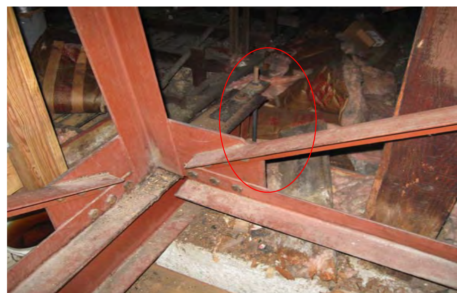
Photo 8 – Tie rod at end of steel beam
