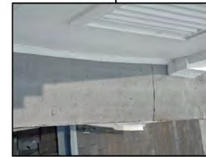
Fiberglass skirt and built-up roofing
