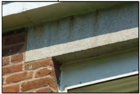
Granite lintel- sandblasted and stained
