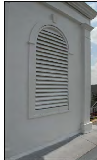
Louvered windows at East and West elevations
