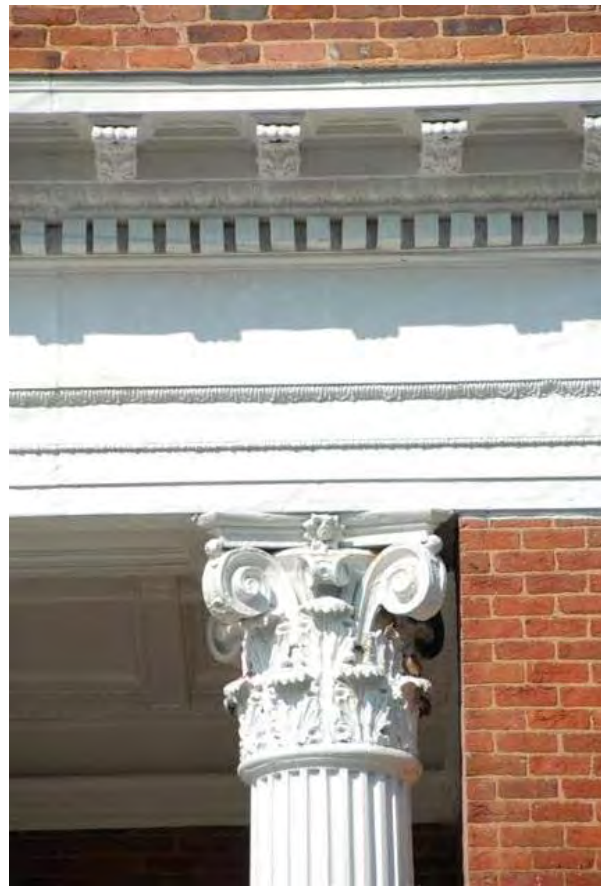
The Corinthian Capital is completely made out of thin sheet metal
