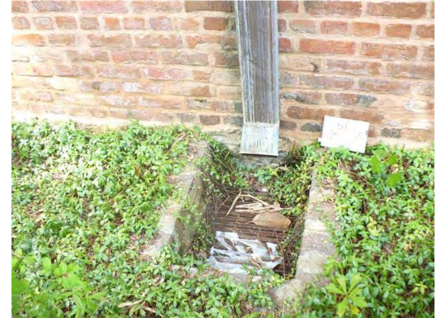
Area drain next to building foundation
