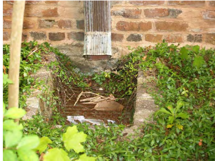
1- Roof Drain Discharge at Grate
