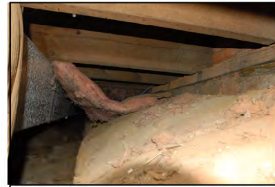
Compacted soil between mechanical duct trench and exterior foundation wall
