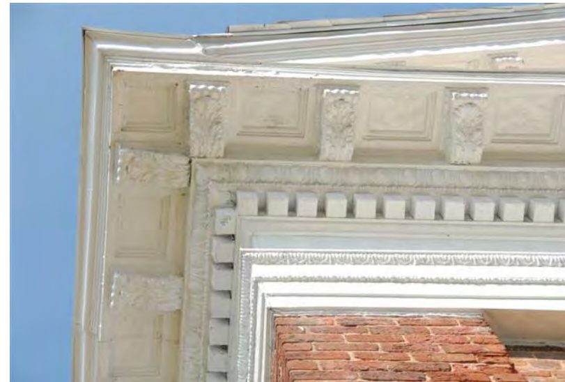
Thin sheet metal cornice and entablature at east gable
