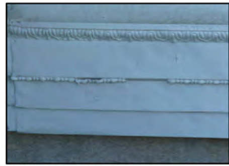
Metal entablature repaired with caulk
