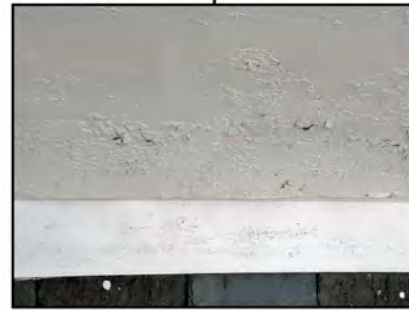
Skirt flashing at North side of tower base
