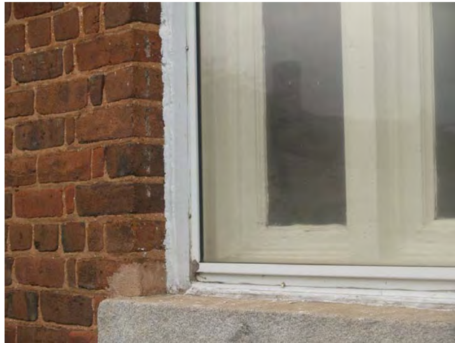
16 Exterior Storm Window
