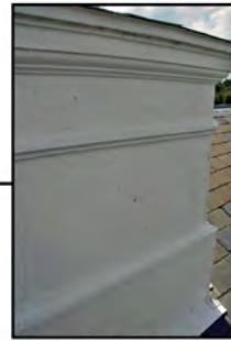
Northside at tower base looking east
