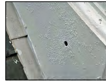
Original metal base of tower with hole
