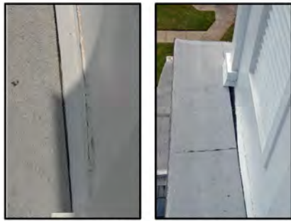
Fiberglass skirt and base at built-up roofing
