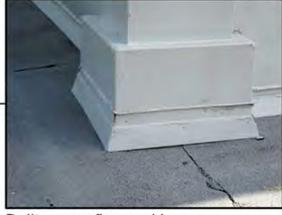
Built-up roofing and base
