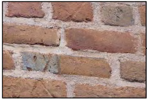
Scratched/ scored masonry
