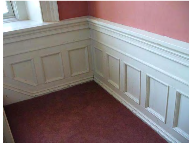
Carpet and wainscot in stairwell
