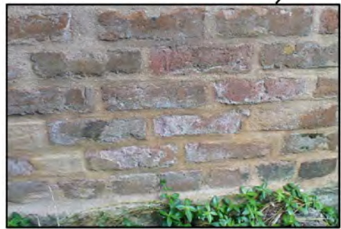
Efflorescence
