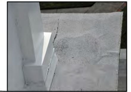
Built-up roofing surface over tower base
