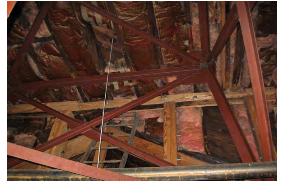
Photo 9 – Additional wood framing members for floor support
