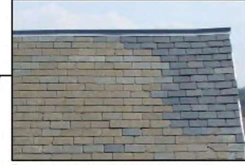
Recently installed black slate replacement tiles at West end of roof
