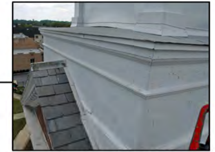
East side, slate roof eave and tower base flashing
