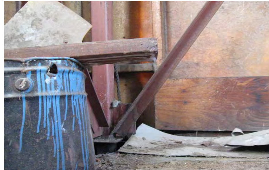
Photo 7 – Transition between lower and upper steel frames
